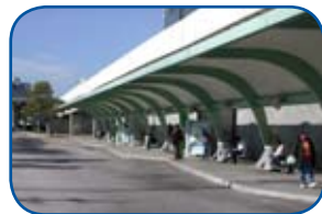
Extended bus platform with assigned berths on Miami-Dade Transitway
