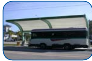
Single length platform on Miami-Dade transitway
