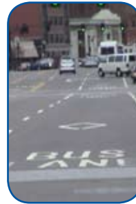
Pavement markings—Boston Silver Line
