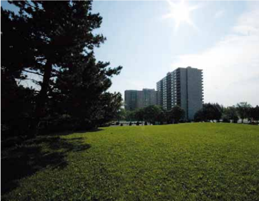
Tower blocks will be refitted in the Mayor's Tower Renewal project
