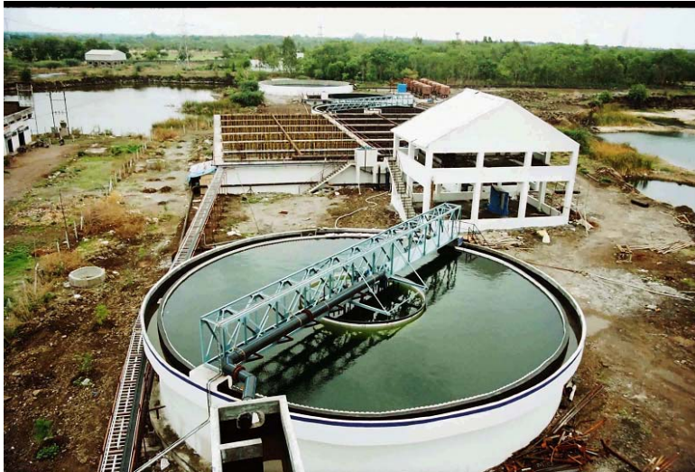
Primary Clarifier (Capacity 9360 CMD)
