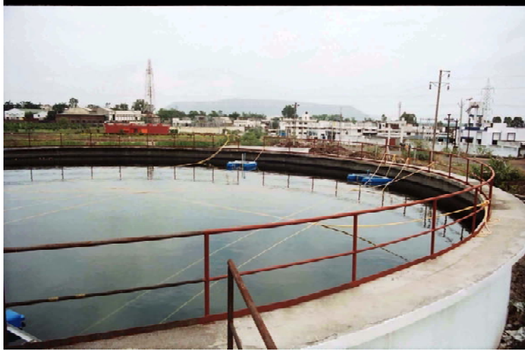
Primary Clarifier (Capacity 9360 CMD)
