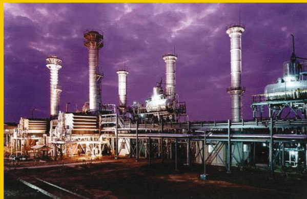
Figure 2.8 • CHP plant at Arvind Textile Mill, India
