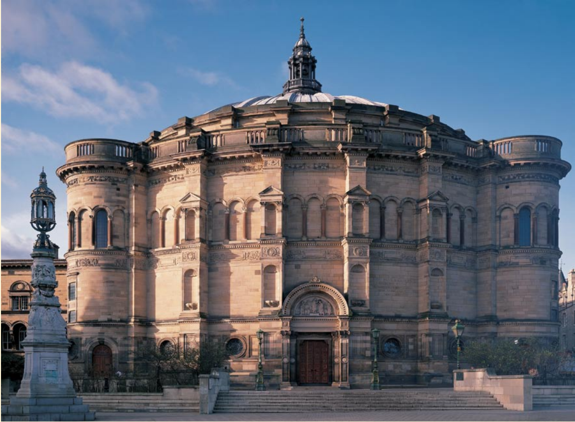
Source: GE Energy
