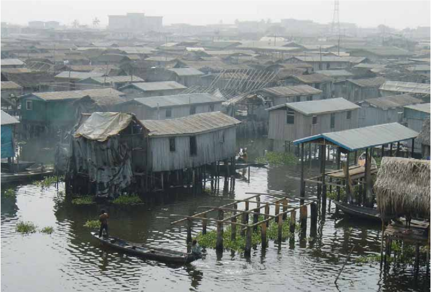
Homes in the low-lying area of Bariga are under threat from rising sea levels
