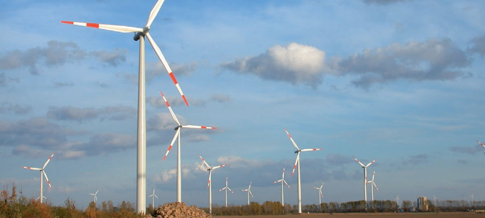
Wind park in Germany, Photo: Dietmar Putscher
