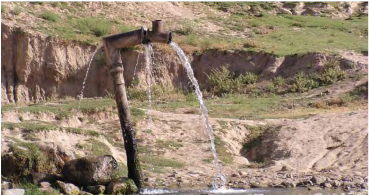
Irrigation system in need of upgrade in Central Asia, R. Everitt 2009.
