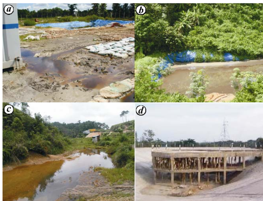
Figure 1. a , Drill cutting fluid due to exploration of fossil fuels. b , Stored in valley with high density poly ethylene lining. c , Leachate through hill crevice. d , Concrete leachate collection and treatment system facility at Masimpur, Cachar, Assam.
