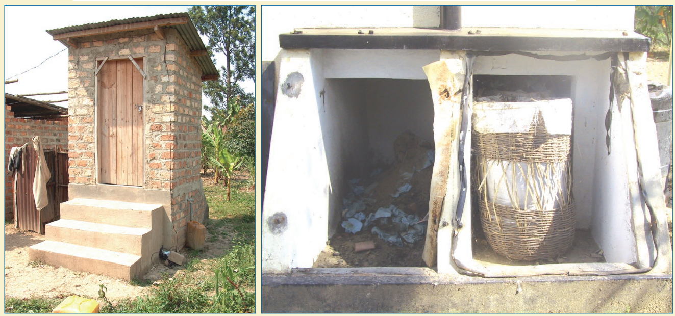
Figure 3: Ecosan toilets in Kabale with a view inside the toilet chamber
