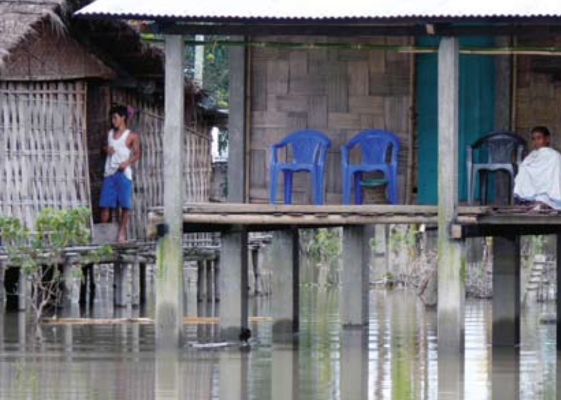
Two types of chang-ghar (house on stilts of the Mishing community) in Matmora: left, the original design of bamboo and wood; centre, wealthier households invest in concrete to make higher stilts.
