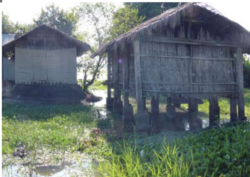
Traditional Assamese houses are built on an elevated platform (left) with a separate granary built on stilts (right).
