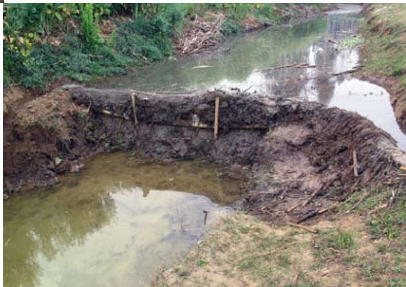
Single earth dam built by an individual household for irrigation of paddy in Taokong, Yunnan, China
