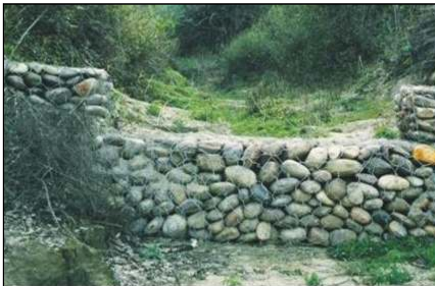
Crate wire with loose boulders
