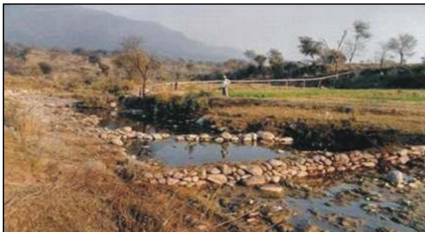
Drain line treatment with stone wall
