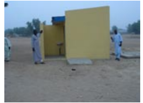
Public Toilet with privacy wall and handwashing facility
