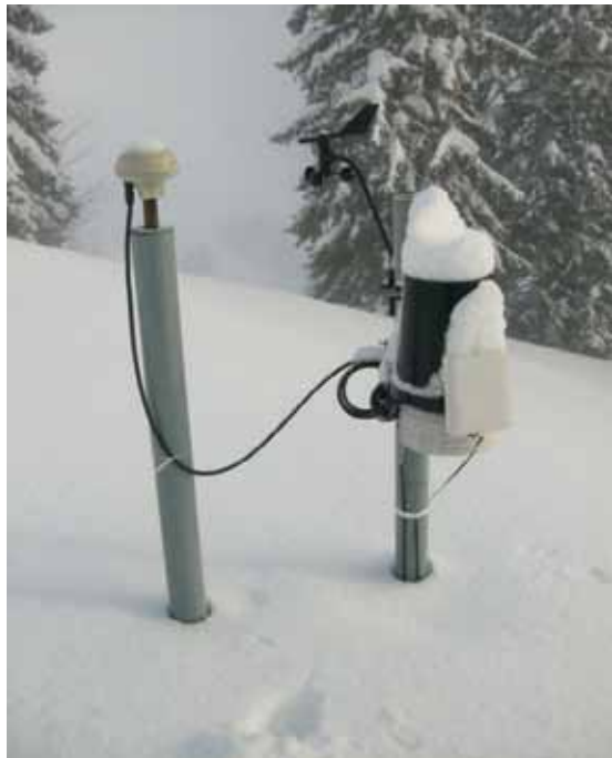
Figure 4: Winter impression at Aggenalm Landslide. The picture shows a Novatel PDGNSS sensor and the weather station.
