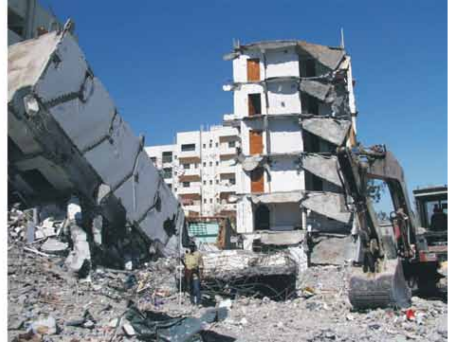
Figure 1: Examples of buildings affected by the 2001 Gujarat earthquake: (Left) heavily damaged residential building, (Right) multi-storey building that has fallen on one side (Bhuj, India) (Image courtesy by M. Markus, 2001)
