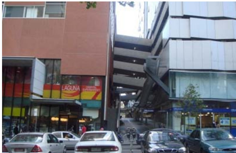
Fig. 2. Flying bridges over the street linking tow buildings in Melbourne-Australia (by the author)
