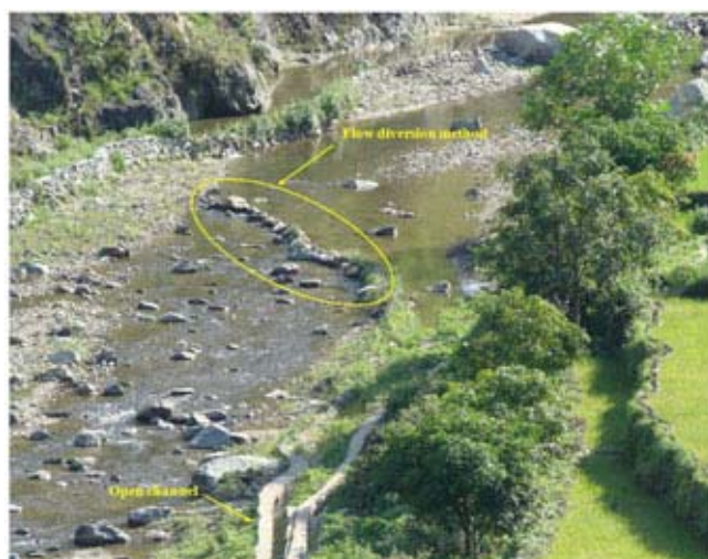
Figure 6. Photograph showing the stream water diversion technique.
