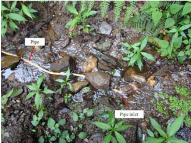
Figure 8. Tapping natural stream water using flexible pipe.
