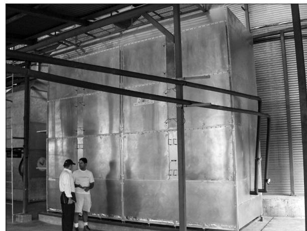
Figure 1: Industrial solar coffee dryers installed at the Montes de Oro Cooperative, Mirimar, Costa Rica. Each tower contains rotating trays on which coffee is placed for drying. Heat for drying is derived from exterior-mounted solar hot-water collectors as also for the gasification of coffee parchment
