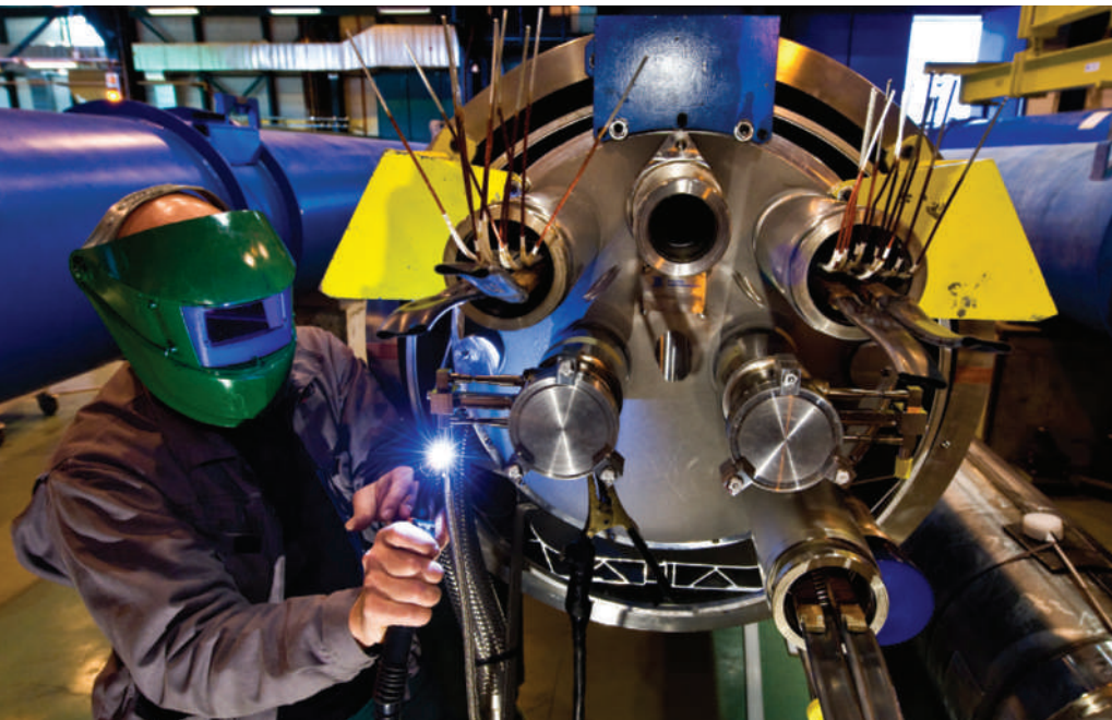
It took months to repair magnets that were damaged in a major accident to the LHC in September 2008.
