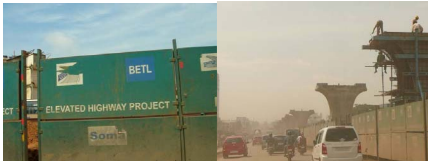
Photo set 3.4: Views of elevated highway construction in progress
