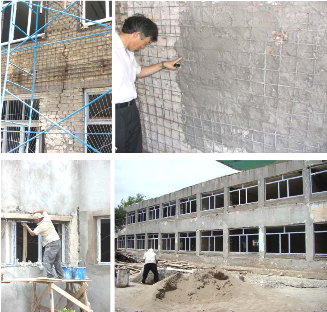
Figure 4.16: School building during retrofitting (Tashkent)
