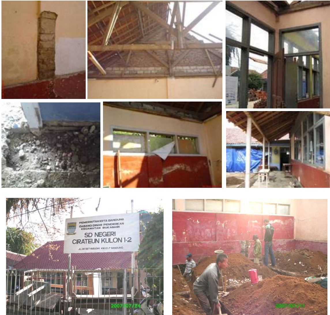
Figure 4.10 Existing structural conditions
