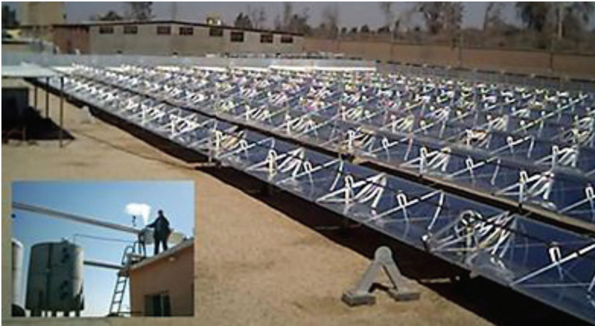
Figure 11 Parabolic trough field, El NASR Pharmaceutical Chemicals, Egypt (Weiss and Mauthner, 2010)
