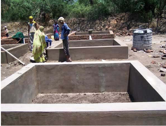
Construction of Compost Pits
