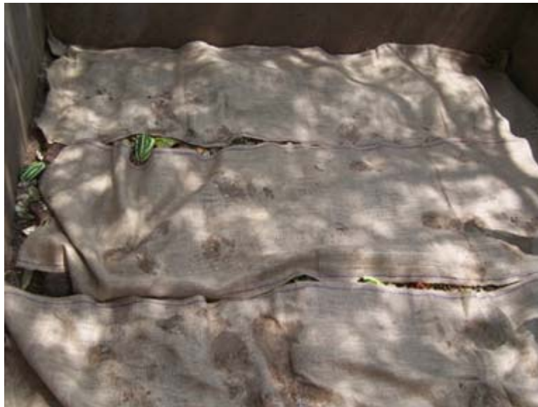
Covering with Jute Sheet after sprinkling of water
