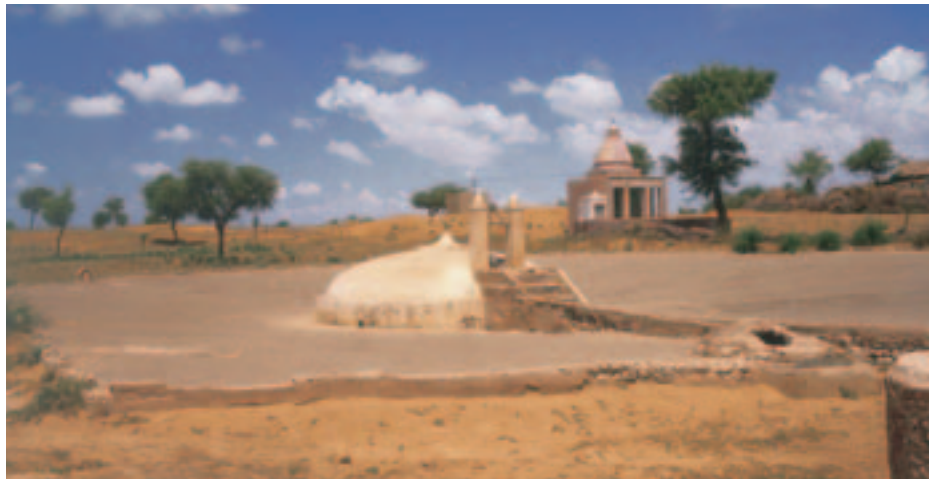
An upturned cup on a saucer! An ingenious system to harvest rainwater on an artificial catchment, called Kundi, found in desert state of Rajasthan. With one hectare of land, and 100 mm of rainfall, one can harvest 1 million litres of rainwater.
