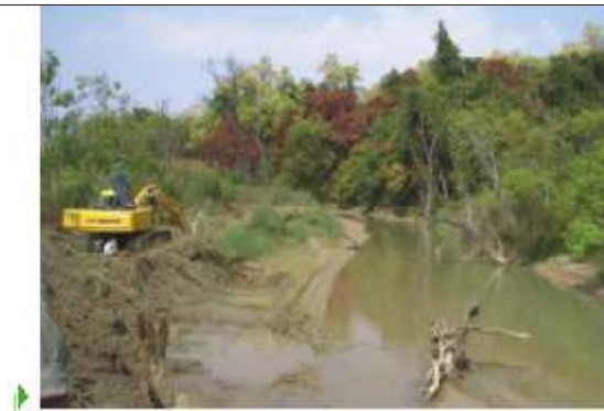
Desilting operation is on using modern machine in DTR
