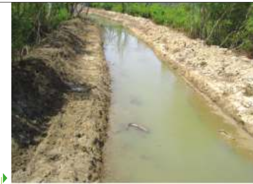
A desilted water channel in DTR
