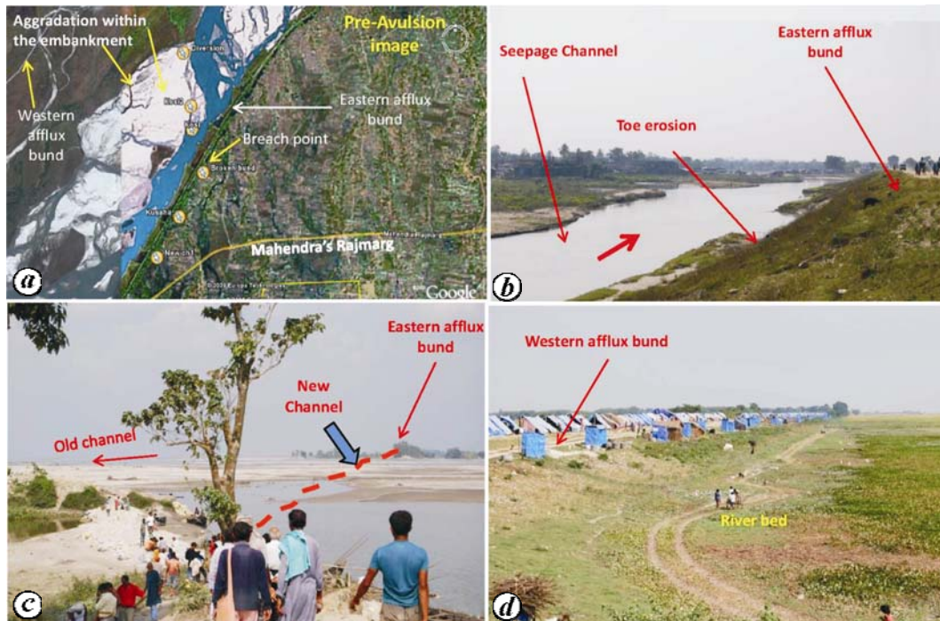
Figure 2. a , Google image showing the course of the Kosi River before avulsion and the breach point at Kusaha; b , Part of the eastern afflux washed away after the breach and the river avulsed towards the east; c , Seepage channel outside the eastern afflux bund causing significant toe erosion; d , The western side of river bed and the afflux bund – river bed is 4–5 m higher than the adjoining flood plain.
