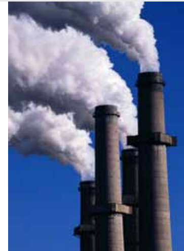
emissions from coal-fired power plant
