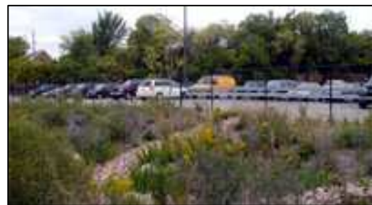
A rain garden absorbs toxins in runoff from an adjacent parking lot in Milwaukee
