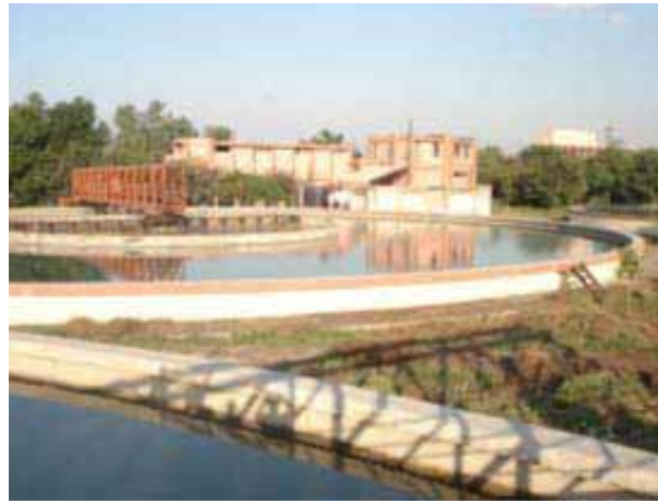
Plate : Clariflocculator at Haiderpur Water Treatment Plant
