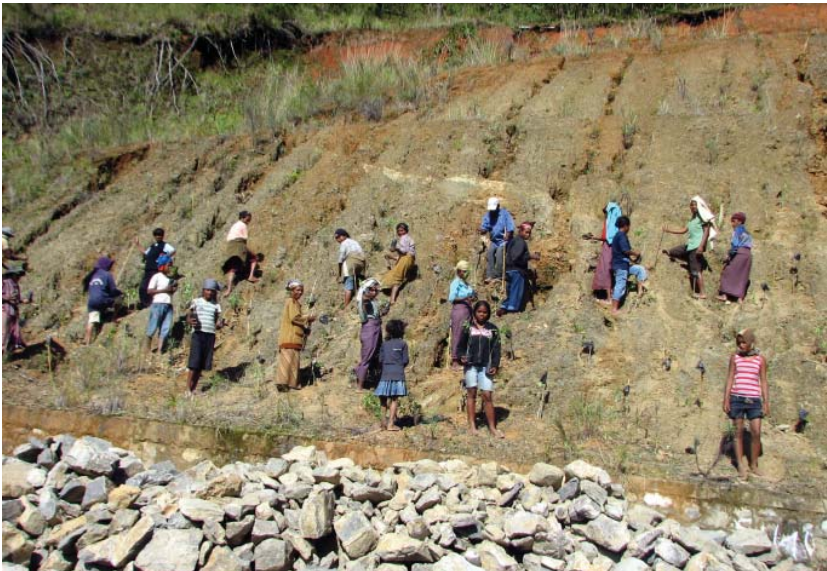
Adaptation to climate change using bio-engineering approach by strengthening slope stability in road construction
