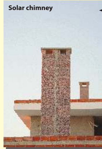
For effective ventilation, specially during humid weather
