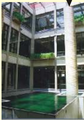
Water moderates harsh ambient conditions around the building
