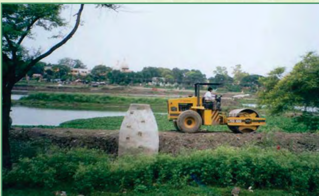
On going work at Rudrasagar, Ujjain
