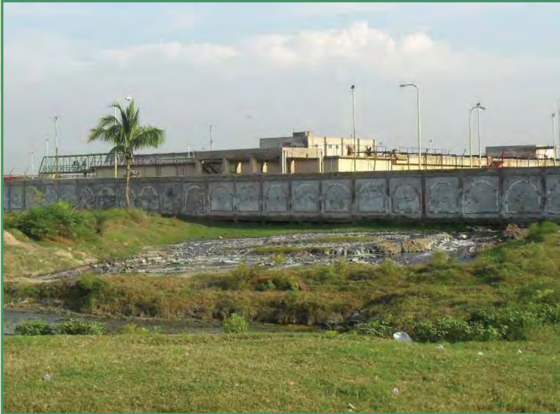
Effluents flowing along the boundary of CETP
