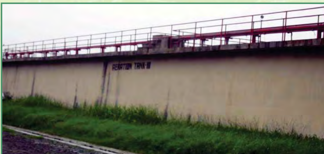
Defunct aerator tank
