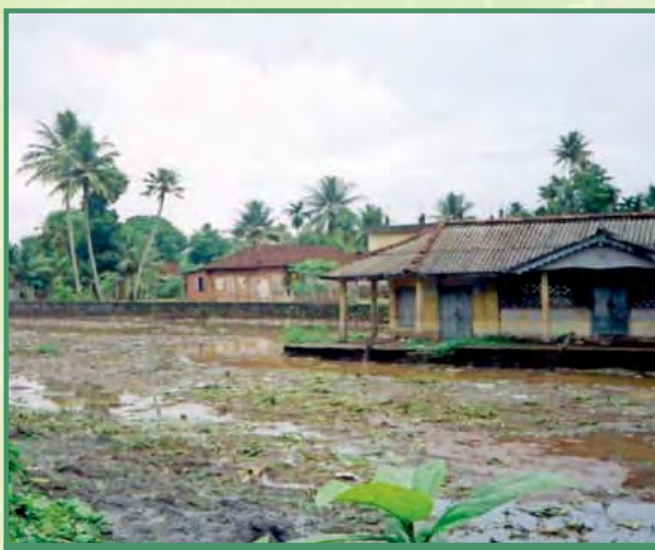
Mundar river, Kottayam after partial work under Ecocity scheme
