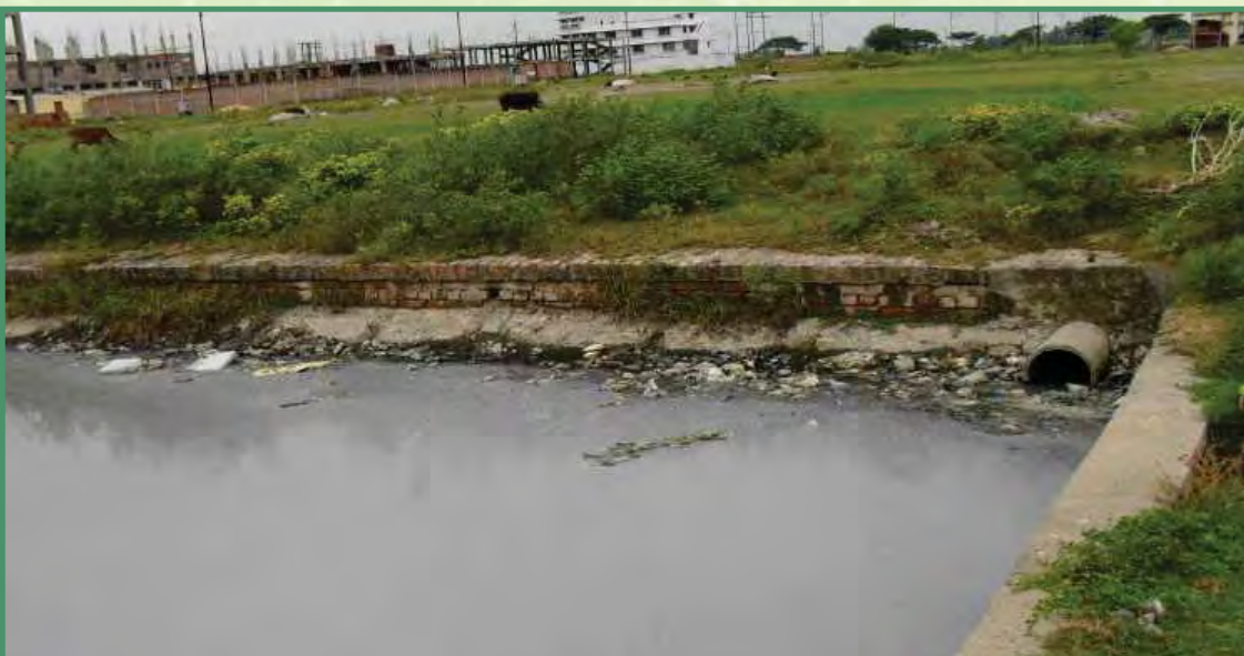
Effluents from the tanneries accumulating in the open
