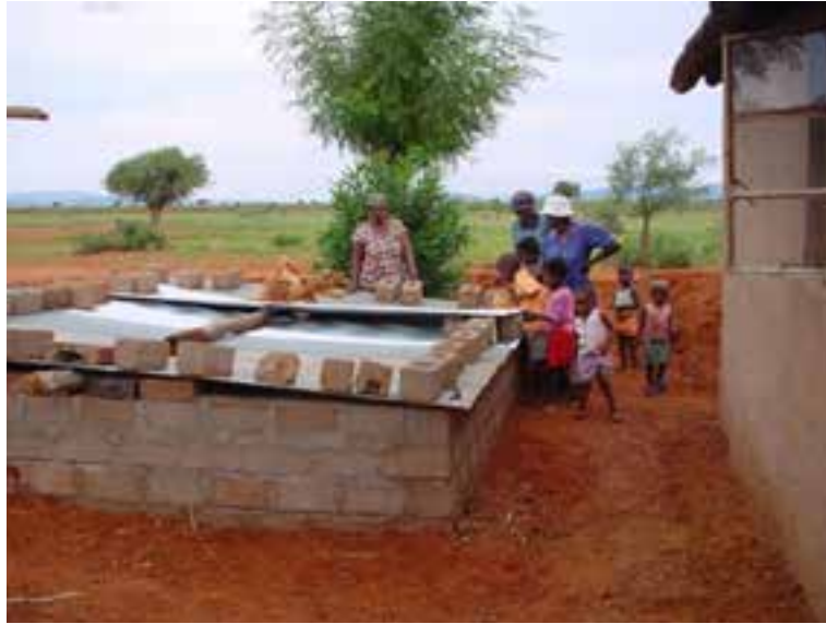
FIGURE 6. Cement block lined underground tank, South Africa.
