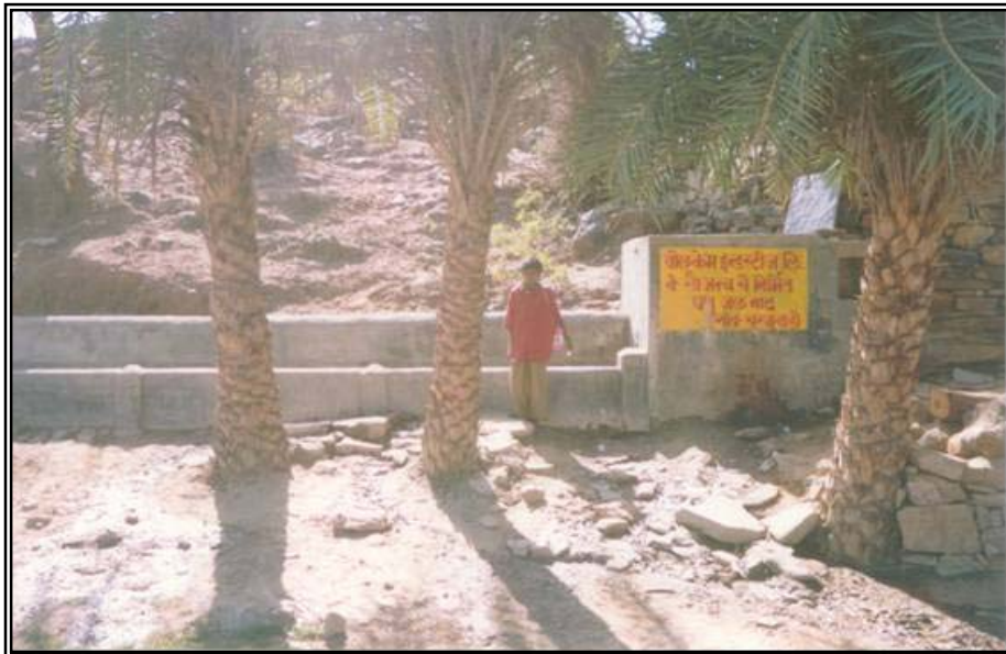
Plate 2.7.6: Construction of Water Tank by Wolkem Industries
