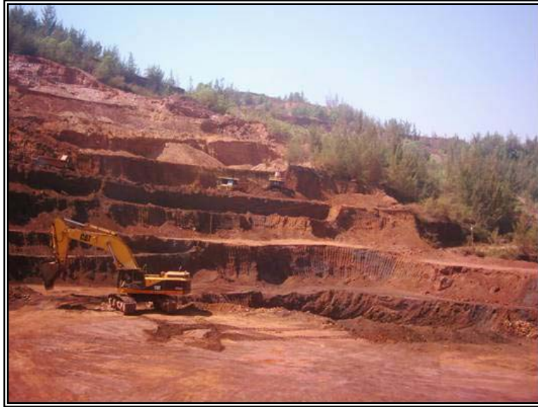
Plate 2.8.1: Environment Friendly Excavation
