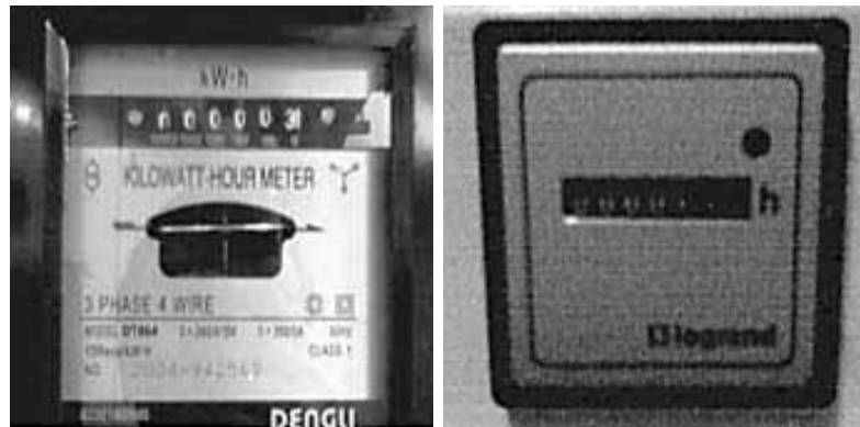
Figures 4 and 5: Monitoring Device Installed – kW-hr Meter & Run-hr Meter, York Air-Cooled System Model: YDAJ98MU7-50PA
