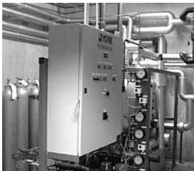
Figure 2: The CO 2 part of the plant and some of the CO 2 cylinders in the background
