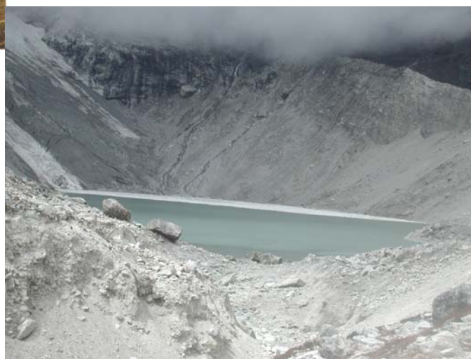
Figure 16: The Dig Tsho GLOF: The site of Namche Hydropower Project destroyed by the GLOF on 4 August 1985 (left) ( Source: WECS). The lake in 2004 (bottom) (Source: WWF Nepal Program)
