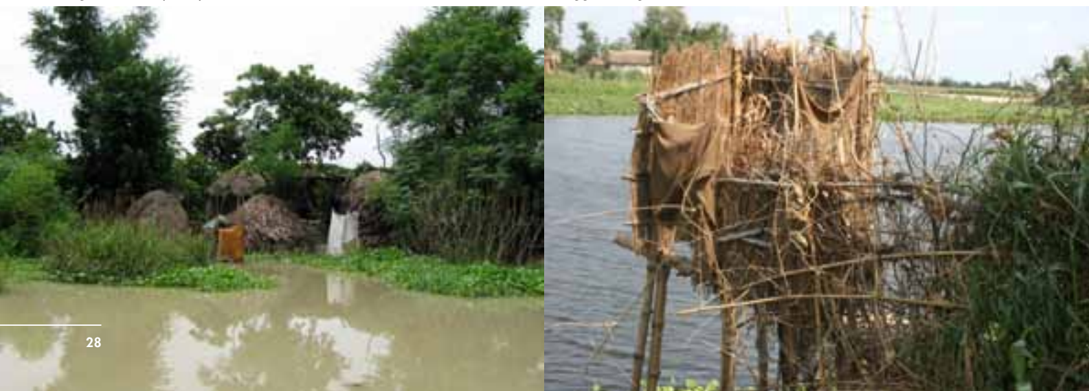
Figure 11: Temporary bamboo latrines constructed in flood-affected and waterlogged villages
