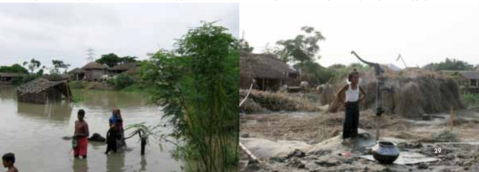
Figure 13: Hand pumps constructed with additional pipes to ensure collection of drinking water even during floods or prolonged waterlogging
