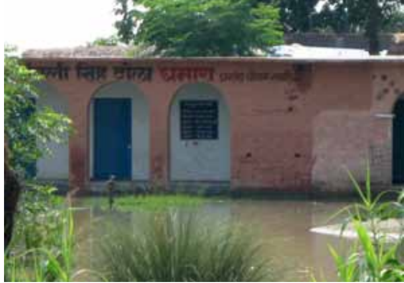
Figure 8: Primary school at Dhamara village closed because of water logging
