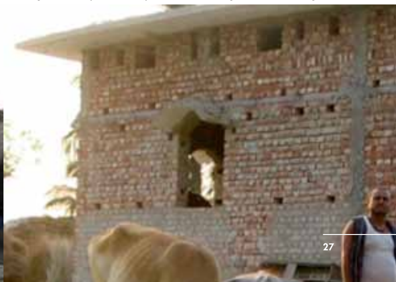
Figure 10: A permanent (pucca) house being constructed using remittances
