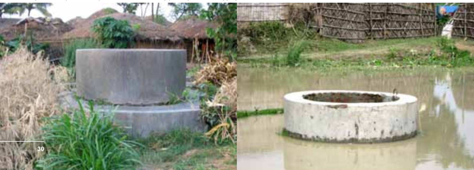
Figure 14: Open masonry well before and during prolonged water logging in Dhamara
