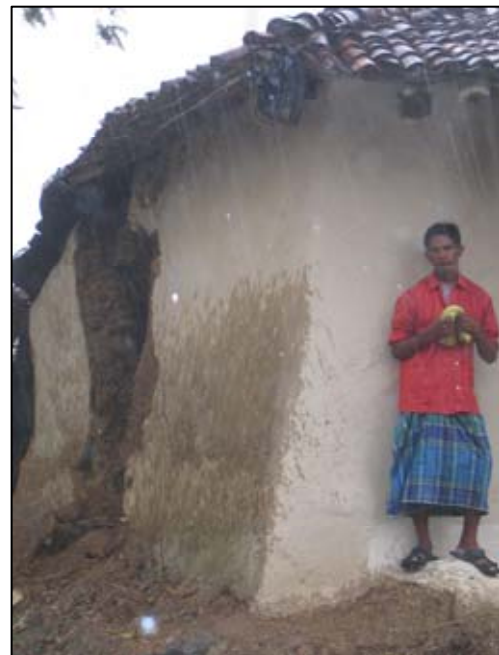
Villagers in Khoddle say that these cracks have been caused by blasting in the project site. Lanco says that the cracks are minor and may have been caused by other factors; no compensation has been provided.
