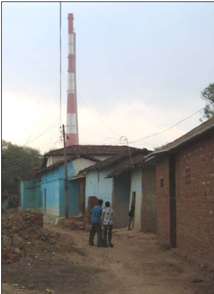
The twin chimneys of the Lanco plant tower over nearby Khoddle
