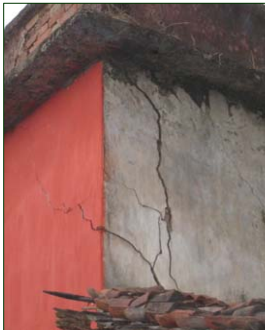
Villagers in Khoddle say that these cracks have been caused by blasting in the project site. Lanco says that the cracks are minor and may have been caused by other factors; no compensation has been provided.
