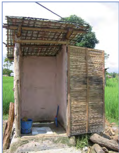
Photo 6: Ceramic pour-flush pan, cement slab, mud plastered bamboo superstructure (Tarai)
