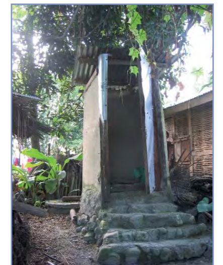
Photo 12: Latrine raised to avoid risk of flooding
