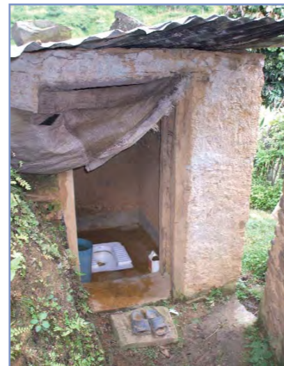
Photo 8: Ceramic pour-flush pan, cement slab, plastered stone superstructure, curtain (hill)
