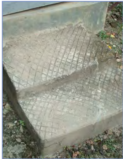
Photo 13: Low steps with cross-hatching to provide anti-slip surface when wet
