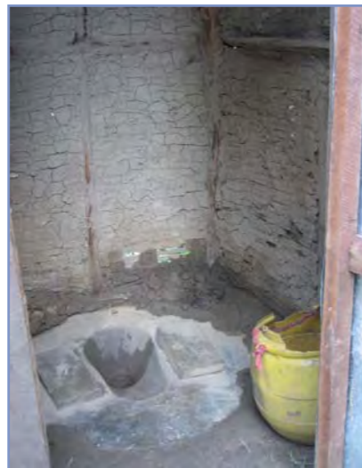
Photo 7: Concrete pour-flush pan and slab, mud plastered bamboo superstructure (Tarai)
