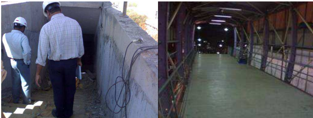
Figure 11 & 12: Pedestrian Underpass under construction and a Skywalk
