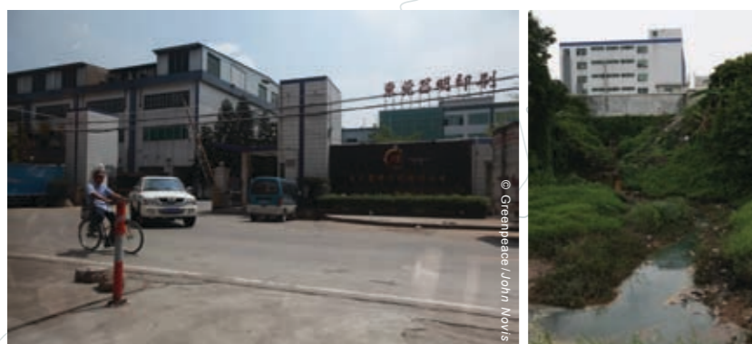
Front gate of the facility
