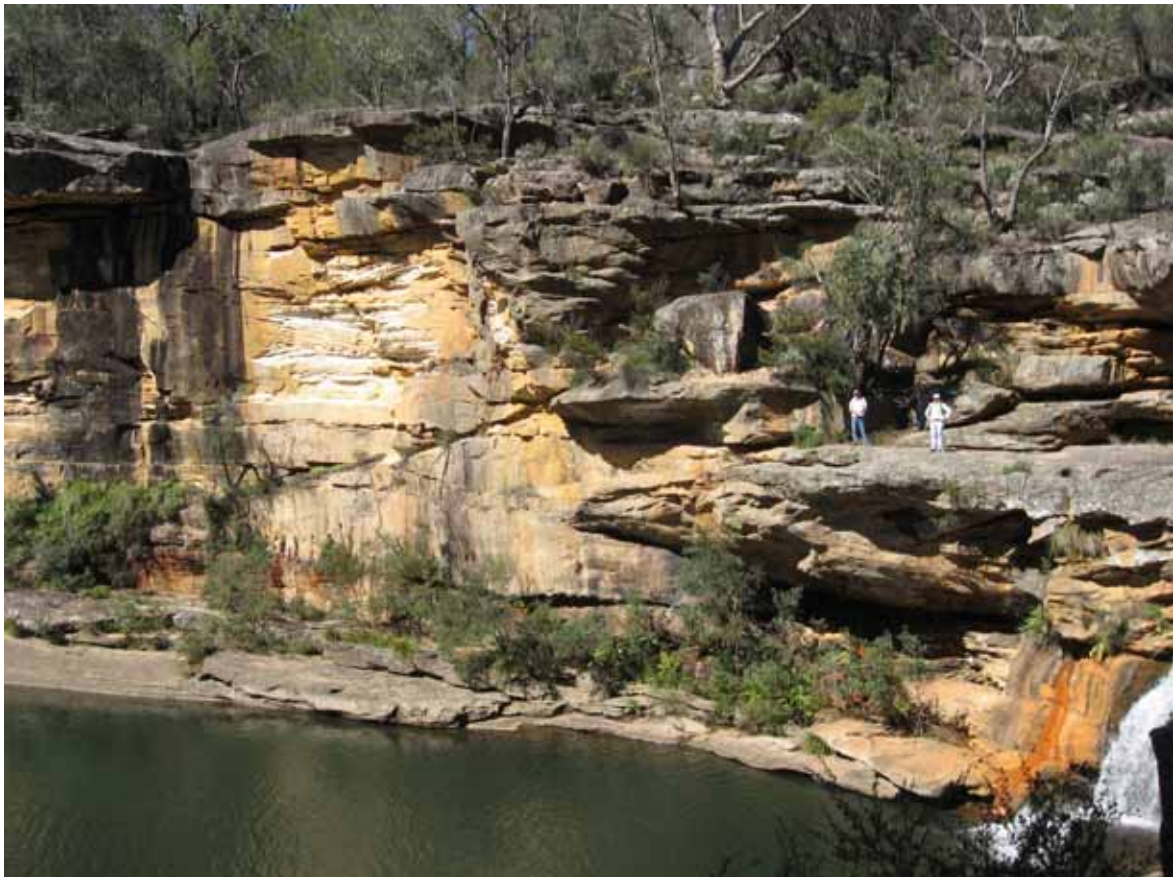
Figure 26: Low Angle Geological Discontinuity in the Walls of Mermaid Pool, Bargo River Gorge
