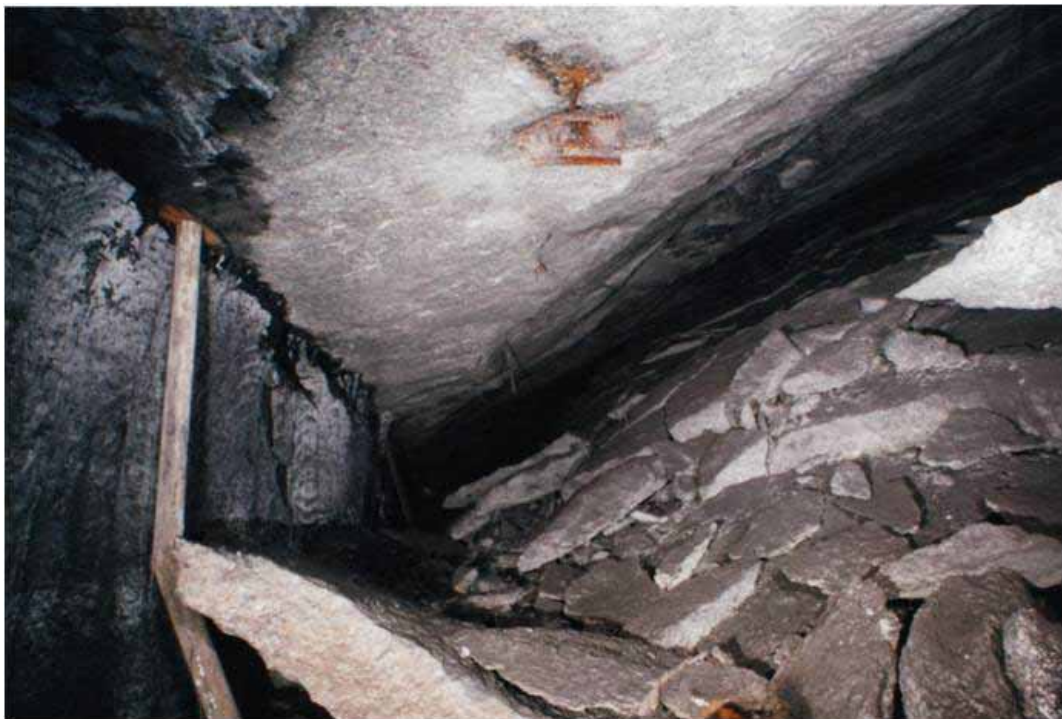
Figure 11: Example of Caving Developing Underground
