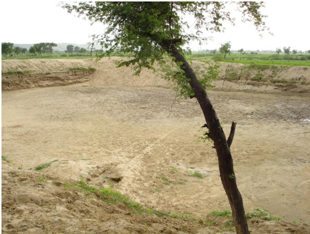
Photo 2.8: Digging a pond through NREGA at Shri Nagar
