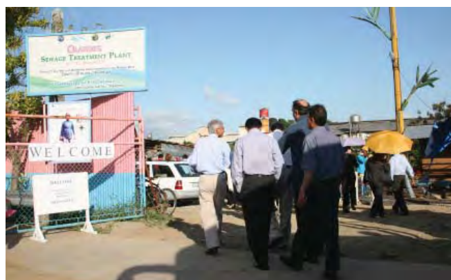
Visit to the ongoing construction of the sewage treatment plant, which is a partnership effort of the city government and Manila Water Company Inc., the private concessionaire
