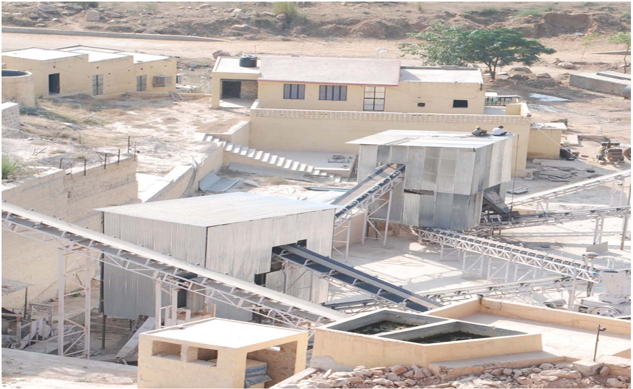
View of the cover on the vibrating Screen
