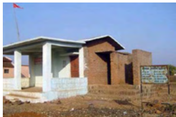
Bus Stand & The half-built public toilet
