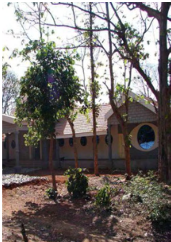
Centralised Accommodation, Banavasi
