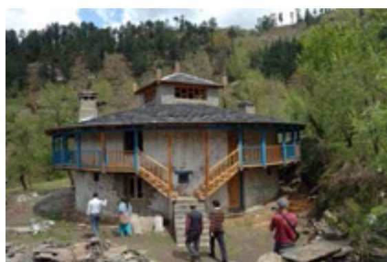
Renovation of Gol Sarai, Naggar
