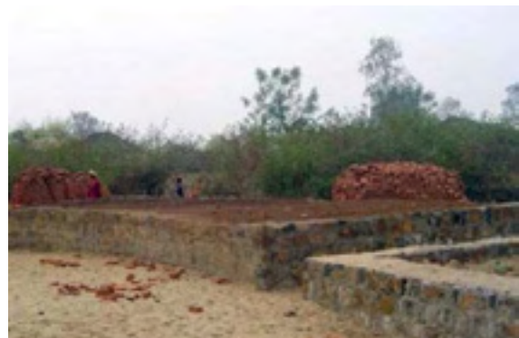
A tourist lodge constructed up to the plinth level
