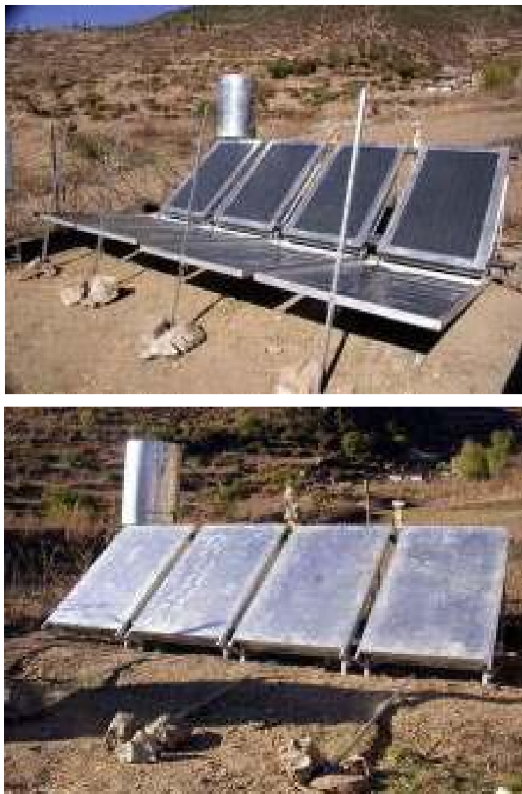
Figure 1-2: SWH system in Nepal having reflectors which acts as cover during night time
