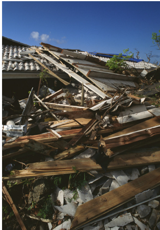
Figure 15 Storm damages by hurricane Katrina.
