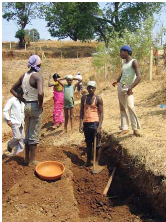
Digging of trenches along contour lines
