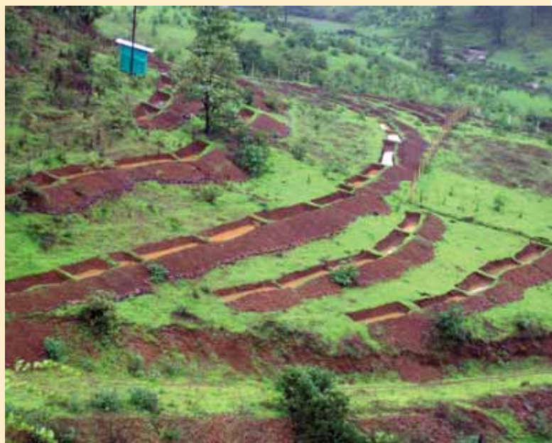
Rainwater impounded in contour trenches
